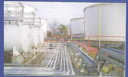
Pipe works for depots and filling stations
