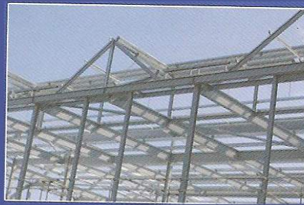
Structure steel work
